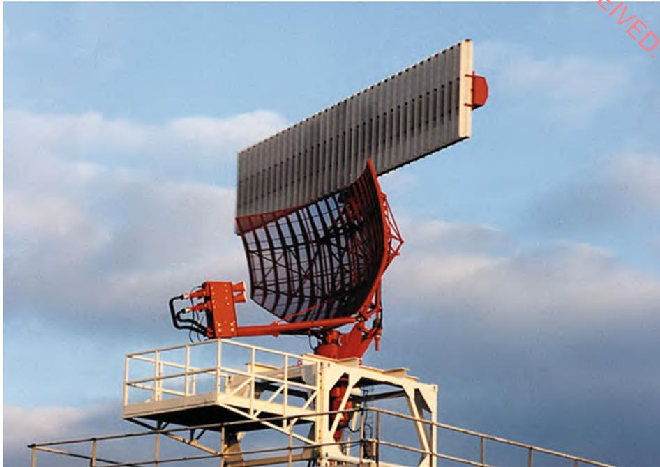
**Figure 4: Primary and secondary co-mounted radar antennas**
